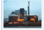
The Public Works Department manages the product (electricity) while Fontana Refuse Disposal Site controls the operation and maintenance of the facility.
