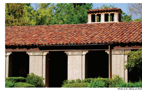
Built in 1900 with natural materials such as clay tile and stucco, the historic Casa Villa is cooled by natural ventilation through top openings such as the one in this photo, and by deep overhangs on the South facade. The preservation and reuse of Casa Villa cost-effectively adapts an existing structure, and serves as an excellent example of how to decrease energy costs through building design and choice of materials.
