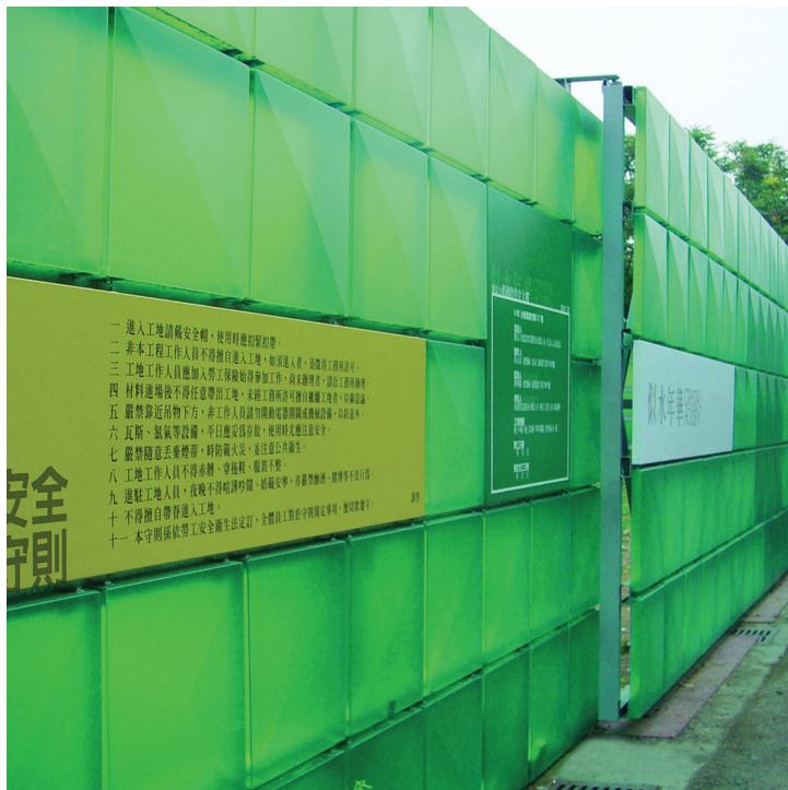
Figure 1 : Construction Fence (2006 IDEA Gold Winner)
